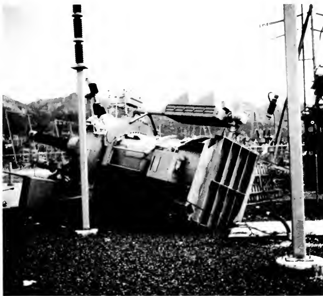
Photo 25. Sylmar Converter Station. Harmonic filter fell over. Anchorage to foundations failed.
